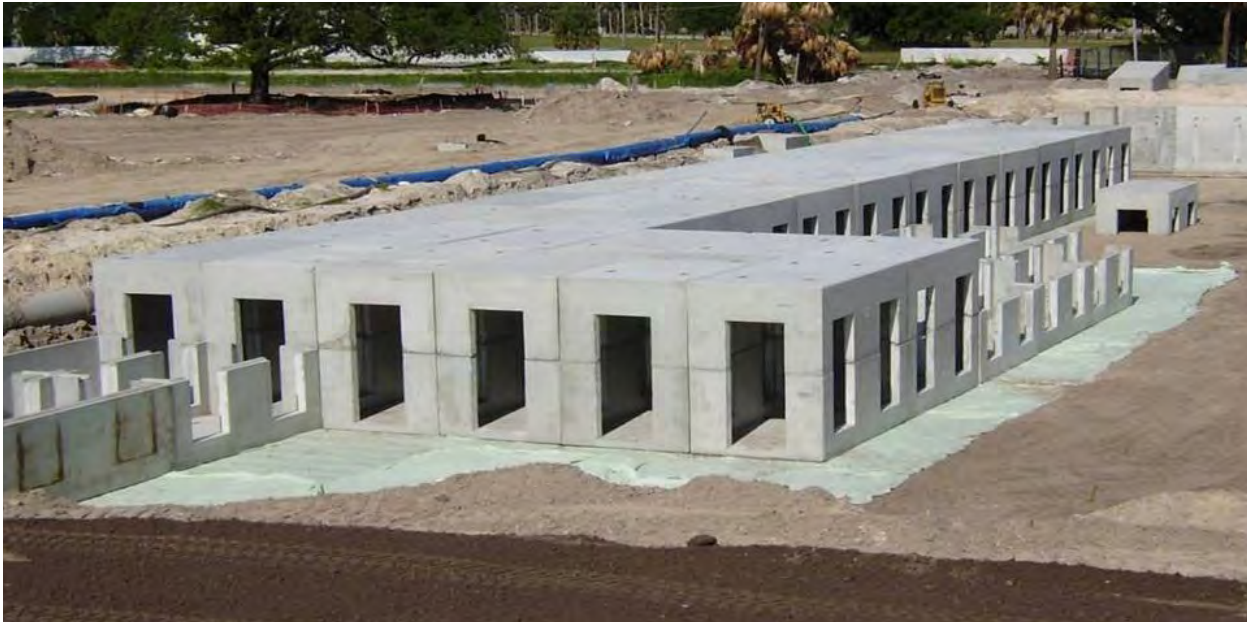
| StormCapture System During Installation Process
